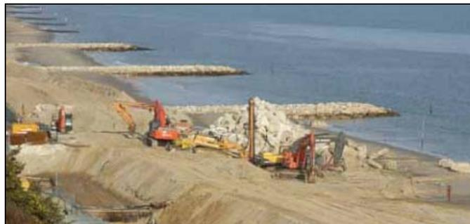
**Photo 9 Stone Groin System under Construction**
