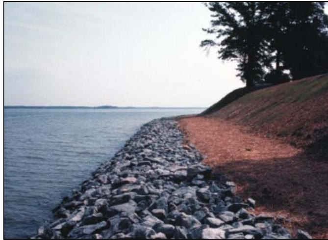
**Photo 8 Typical Riprap Rock Revetment –
