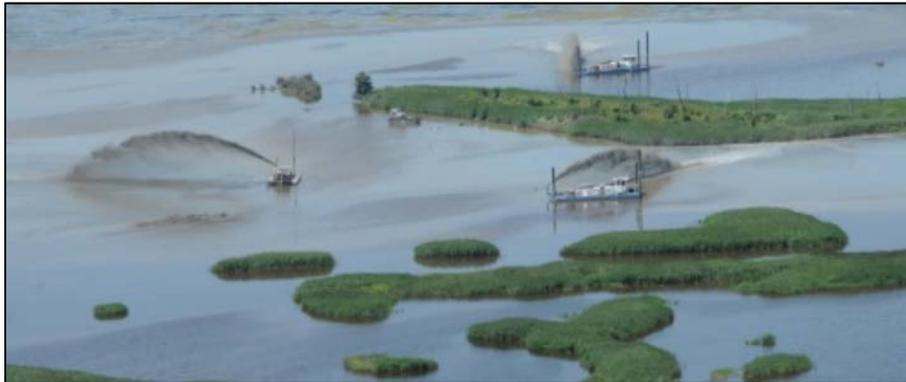
**Photo 2 Thin Layer Placement Construction Underway at Prime Hook National Wildlife (USFWS Website 2019)**
